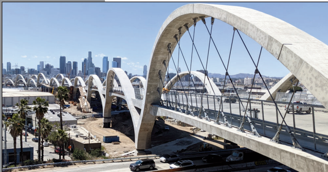
Sixth Street Viaduct, Los Angeles, USA / Customer: COWI North America
